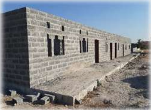
Arise block walls completed.
